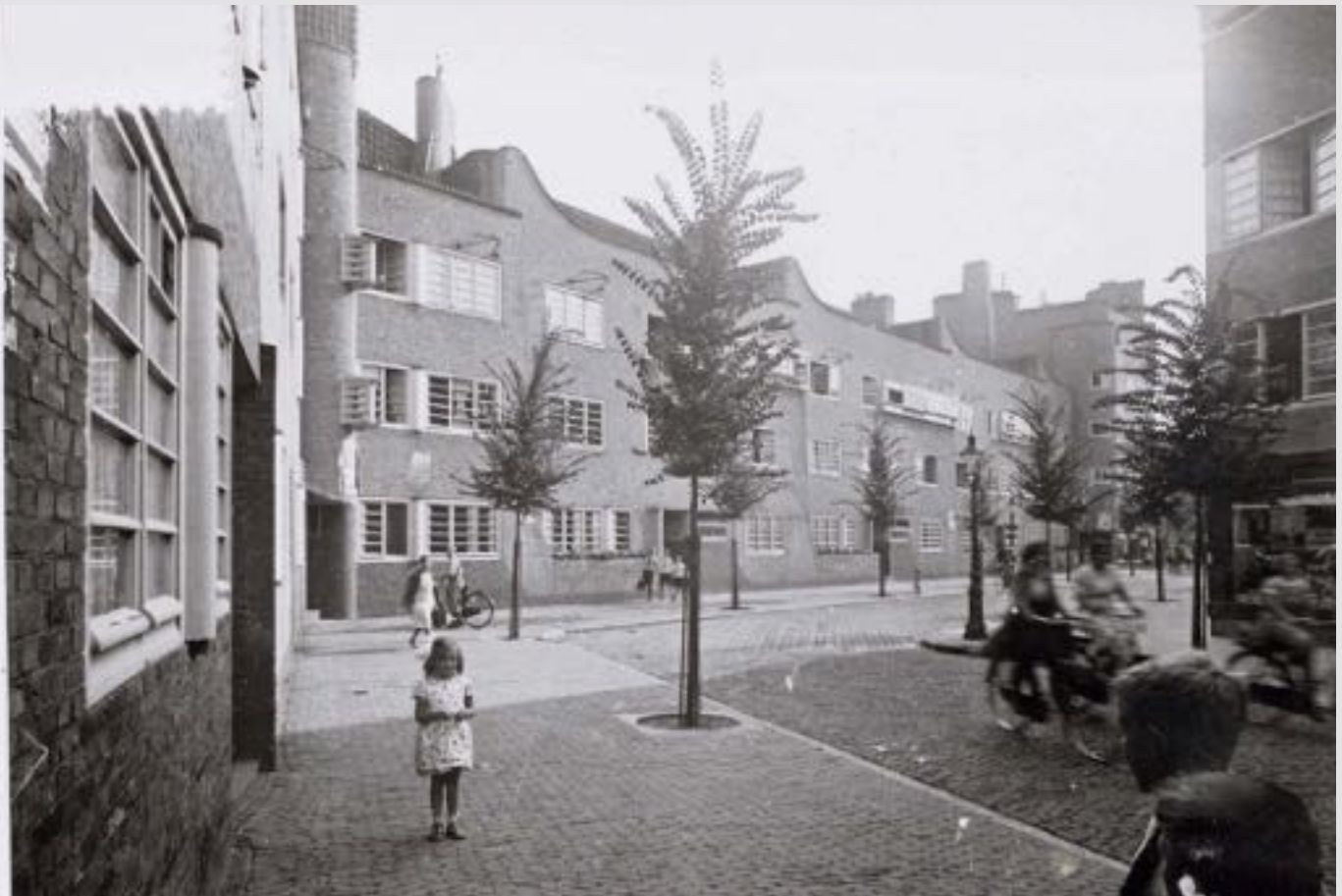
figure 3.29. social housing complex de Dageraad part of the 'Plan Zuid', these kinds of blocks were meant to provide affordable and subsidized housing for working class families in Amsterdam (Stadsarchief Amsterdam, 1932)
