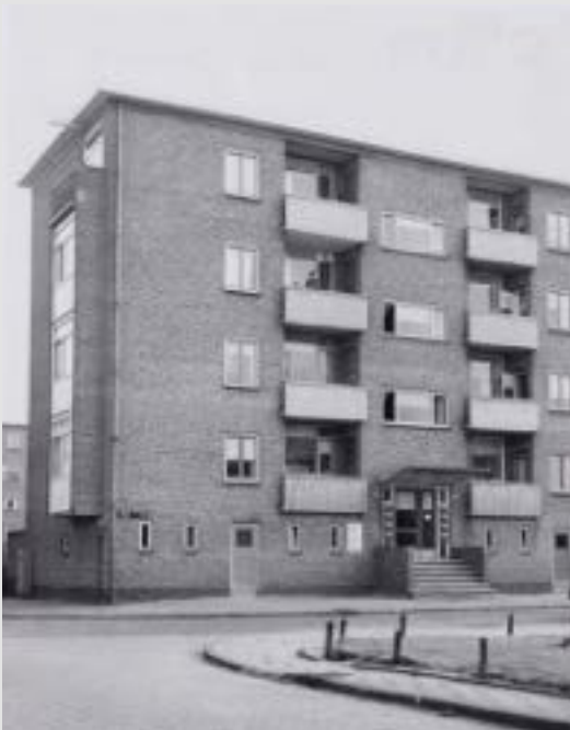
figure 3.32. With the development of the Westelijke Tuinsteden new types of houses were introduced such as this one in Geuzenveld (de Gemeentelijke Dienst Volkshuisvesting / Stadsarchief Amsterdam, 1958).
